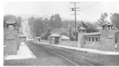
The Oakland Avenue Street, Built by the City of Piedmont in 1910. Looking Eastward.
